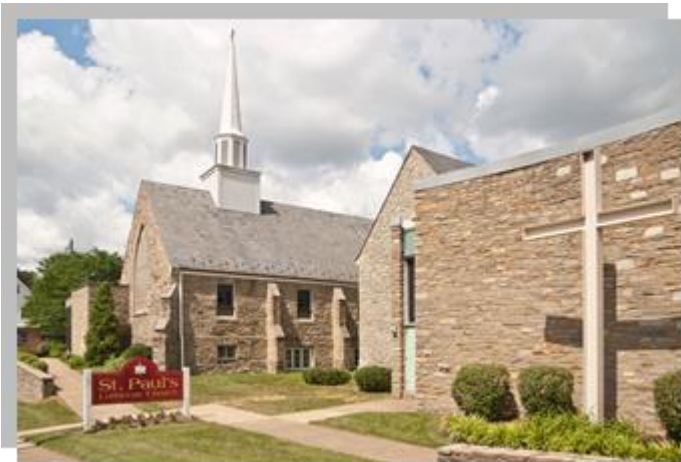
St. Paul's Lutheran Church 120 N. Easton Road Glenside PA 19038
